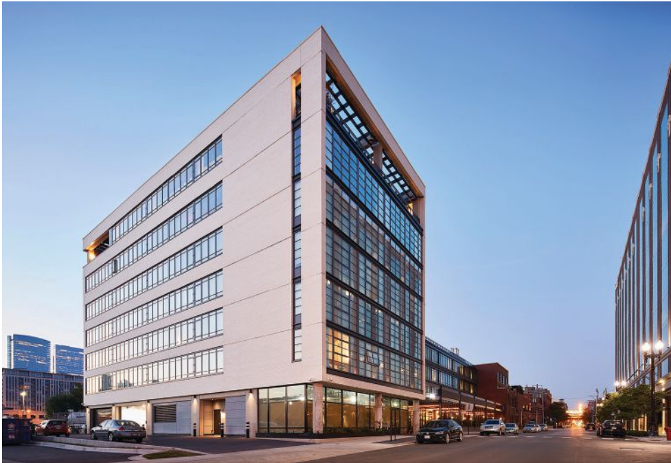
GREC Architects' new project, the Ace Hotel, has opened in the West Loop. The building preserves the existing Fulton Market landmark cheese factory façade on the south side of the building.
